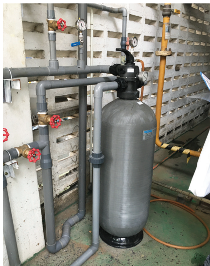
Waterco proposed the commercial grade W400 filter with Glass Pearl media, a filtration solution to maximise the performance of their cooling tower.
