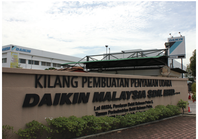
With a total built up area of 7,340 square feet, Daikin Malaysia is the largest air-conditioner research and development (R&D) centre in South East Asia.
